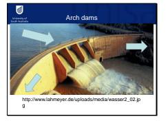
Gravity dams are a simple idea, and aren't necessarily efficient in terms of materials. Arch dams are more elegant than gravity dams for engineering solutions. Whereas the gravity dam relies on absolute weight for holding water back, the arch dam relies on deflecting that force out to the sides, so it's got the advantage of any arch structure. Arch dams can be concave in one or both directions.
