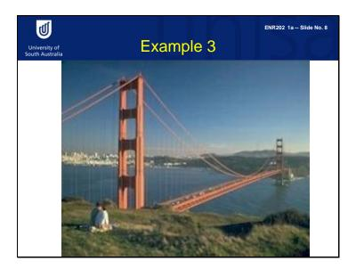
This is a long, cable-stayed bridge. We can have cars and pedestrians on the bridge. The self weight of the cars need to be transferred to the deck of the bridge and then to the ties of the bridge cables. The cables transfer the loads to the tower of the bridge and to the supports of the bridge. Finally, the structure of the bridge transfers loads to the foundation.
