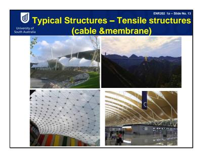
Here we see a tensile structural type. Here we have a membrane and cable structure: membrane and cable (top left), and membrane with cable in two directions (bottom left.) The membrane and cable system may transfer wind load to the foundations. We also have a cable stayed bridge (top right), and a cable truss structure (bottom right), where the cable will only carry tension, and the truss will carry both compression and tension – we will talk more about these terms in later lectures.
