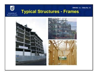
In this image, you can see different kind of structural frame types. A frame means a system of beams, columns and fixed joints between them. After put together, the frame structure may transfer forces and bending moments. We can have concrete framed structures (as in the image on the left), or steel framed structures (top right) or timber framed structures (bottom right).
